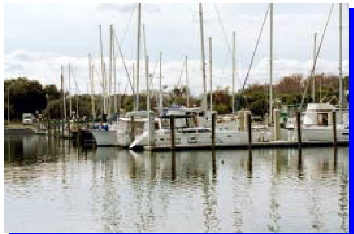
Without continual maintenance of the waterways, shoaling would prevent the use of the waterways by a significant portion of the pleasure craft in the county, such as the sailboats pictured
